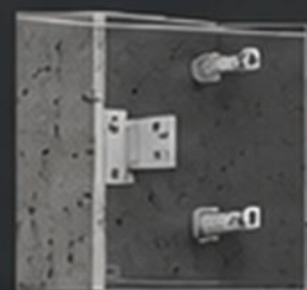
STEP 01 Fix Helping Hand Brackets to RCC Wall
